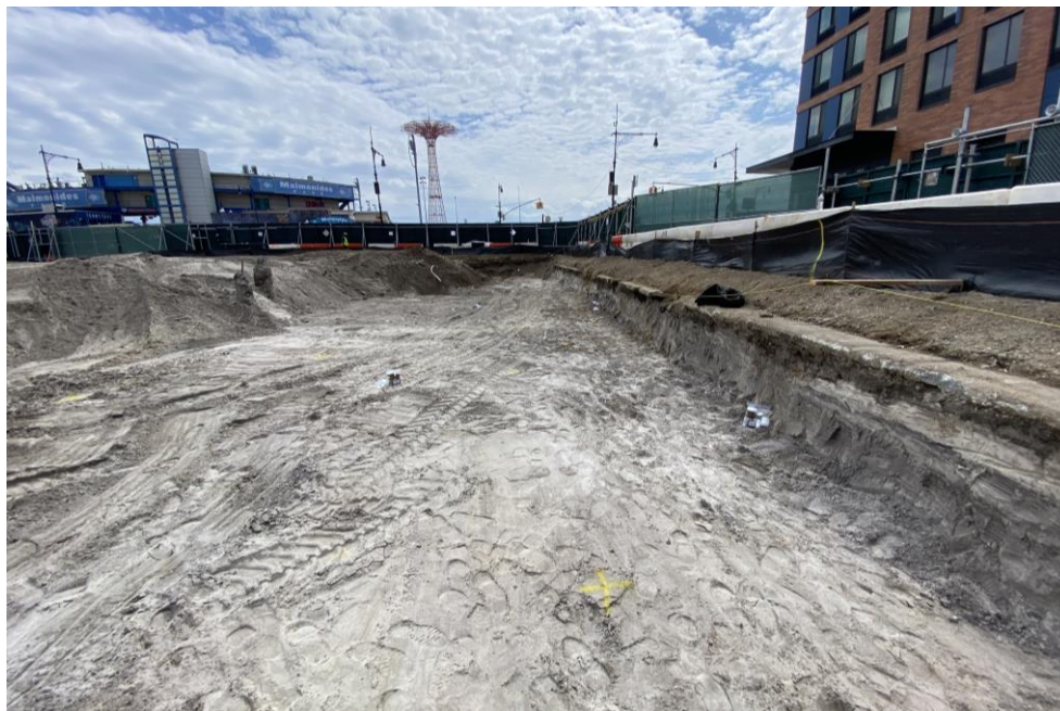
Photo 2: View of remedial subgrade in the western part of the site (facing south).
