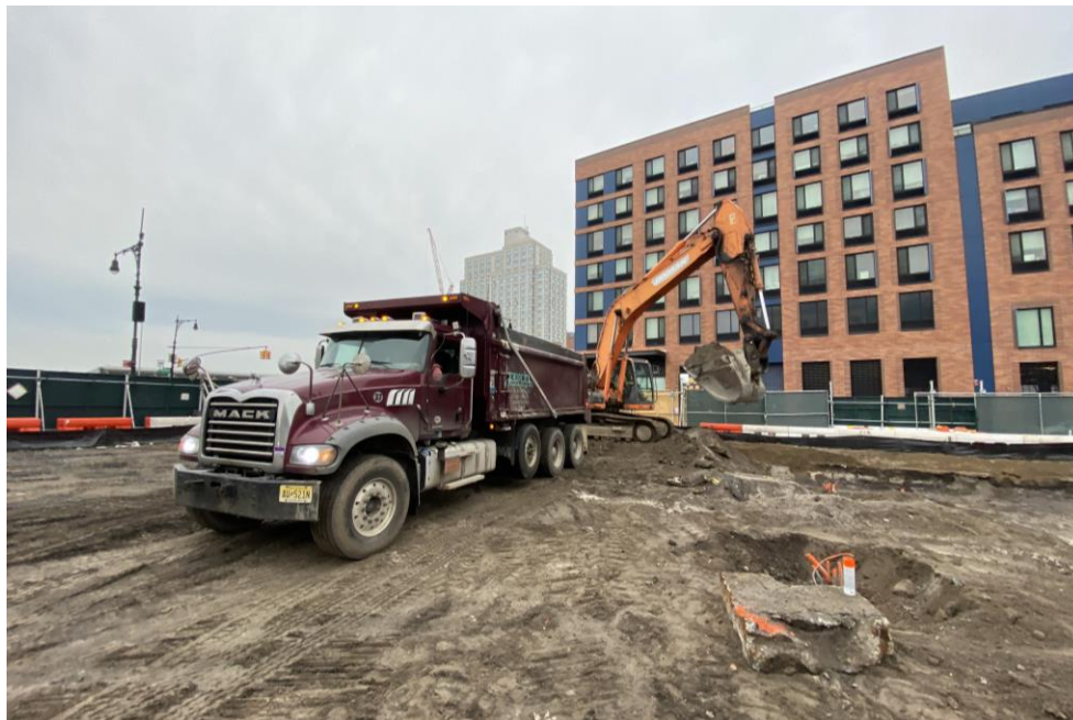
Photo 1: Precise excavating non-hazardous fill/soil in the western part of the site (facing southwest).
