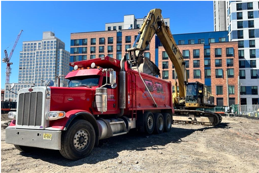
Photo 1: Precise live-loading non-hazardous fill/soil for offsite disposal in the southwestern part of the site (facing southwest).
