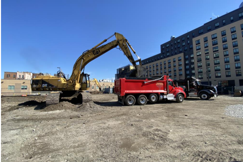
Photo 1: Precise live-loading non-hazardous fill/soil for offsite disposal in the central part of the site (facing northeast).
