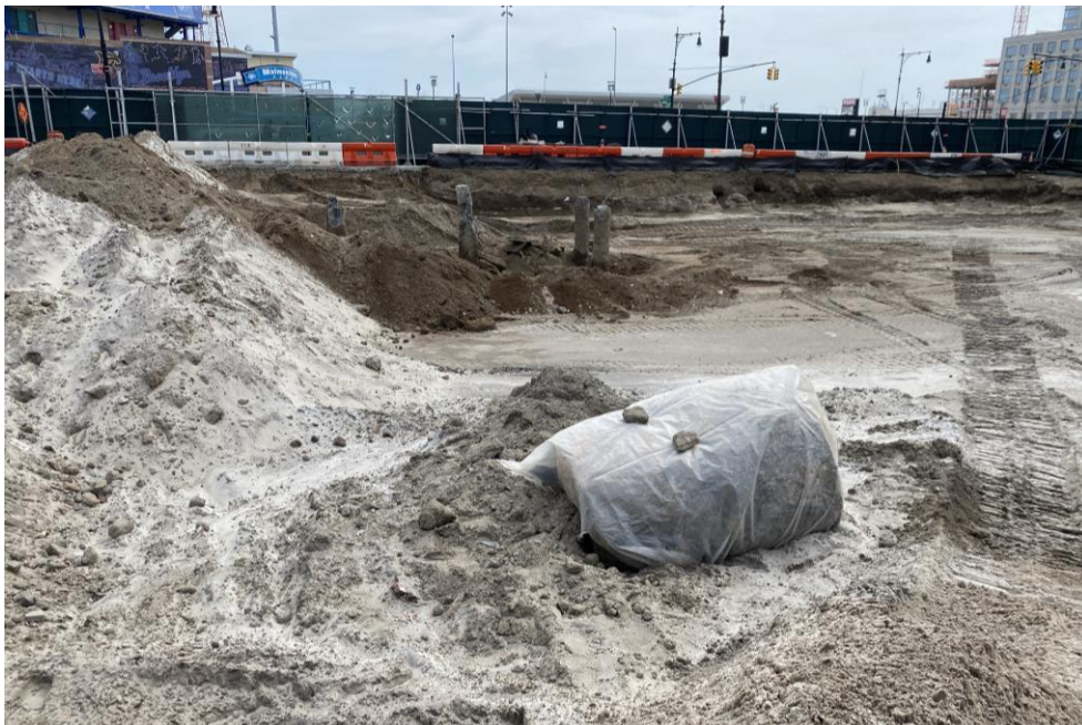
Photo 2: View of uncovered UST in the central part of the site covered with polyethylene sheeting (facing southwest).
