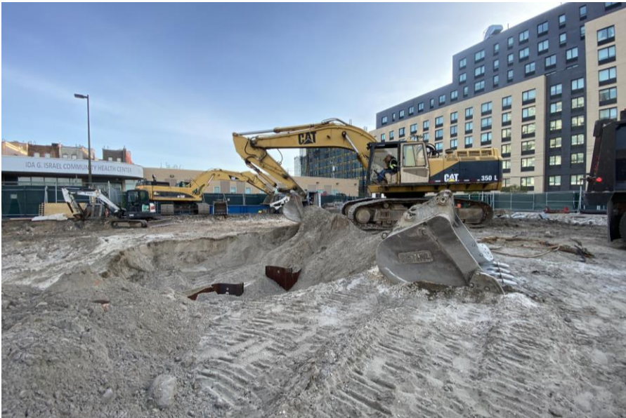
Photo 1: Precise excavating non-hazardous fill/soil for future offsite disposal in the east-central part of the site (facing northeast).
