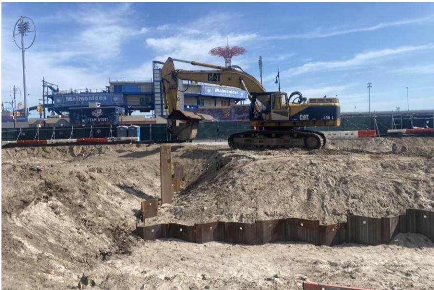
Photo 2: Precise installing sheet piles in the east-central part of the site (facing south).
