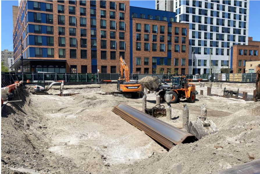
Photo 1: Precise constructing an elevated pad to facilitate sheet pile installation in the southwest part of the site (facing west).
