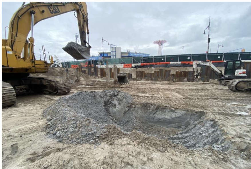
Photo 2: Precise excavating for the dewatering sump in the southern part of the site (facing south).
