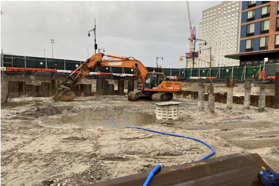
Photo 1: View of the dewatering sump in the southern part of the site (facing southwest).
