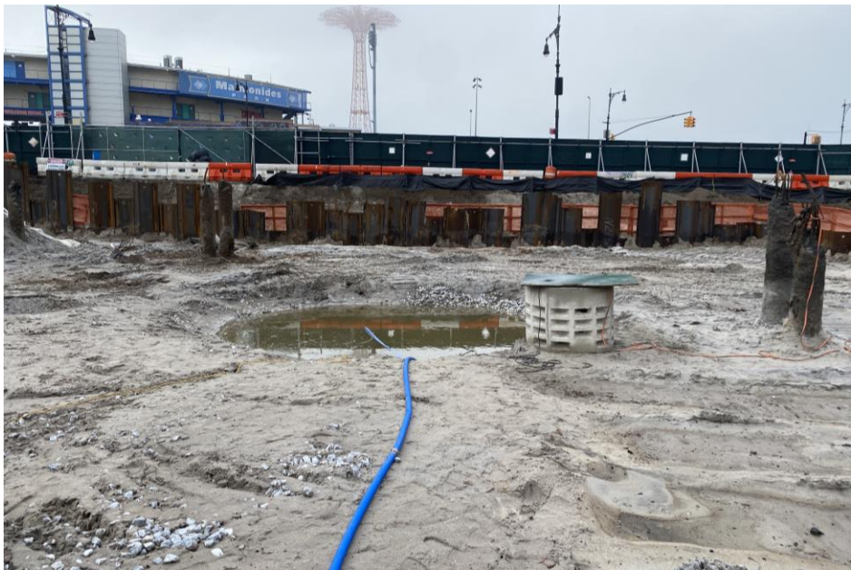
Photo 1: View of the dewatering sump in the southern part of the site (facing south).
