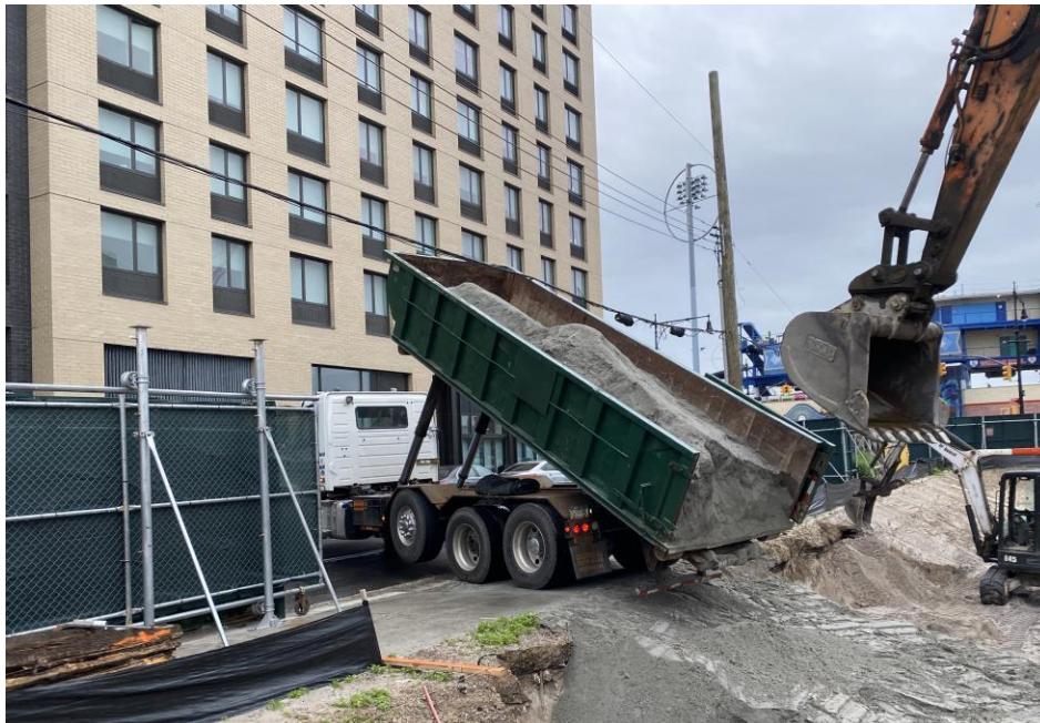
Photo 2: Precise importing pipe sand in the eastern part of the site (facing southeast).
