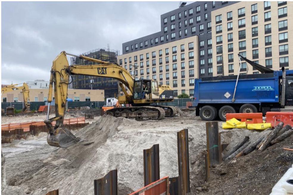
Photo 1: Precise loading non-hazardous fill/soil for offsite disposal in the southern part of the site (facing northeast).
