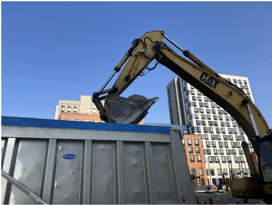
Photo 2: Precise exporting non-hazardous soil/fill for offsite disposal (facing west).
