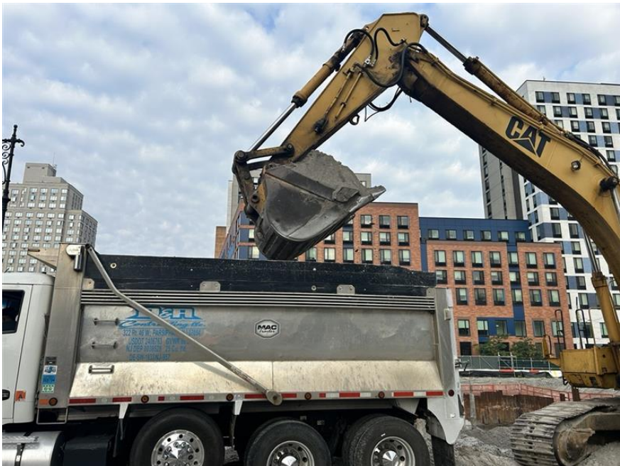
Photo 2: Precise exporting non-hazardous fill/soil for offsite disposal (facing west).
