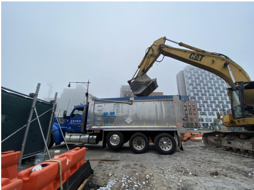
Photo 2: Precise loading non-hazardous fill/soil for offsite disposal (facing southwest).
