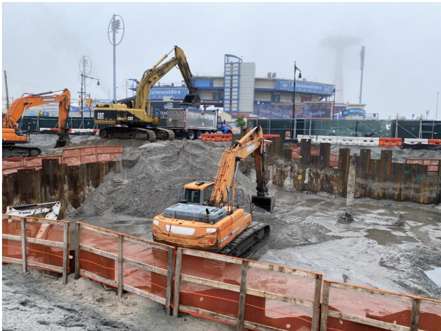
Photo 1: Precise excavating non-hazardous fill/soil in the southern part of the site (facing west).
