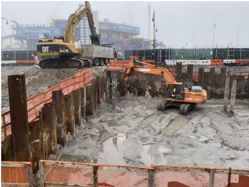
Photo 2: Precise excavating and live-loading non-hazardous fill/soil for offsite disposal in the southern part of the site (facing south).
