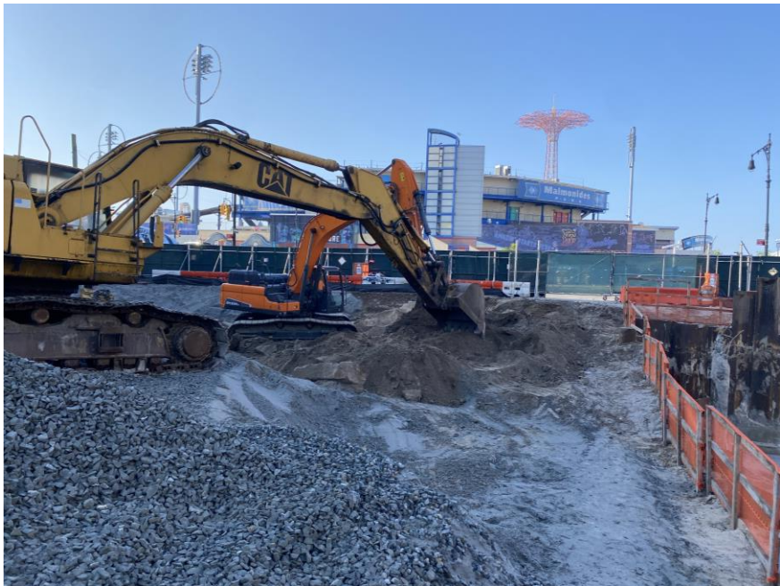
Photo 1: Precise excavating non-hazardous fill/soil for offsite disposal in the southern part of the site (facing south).
