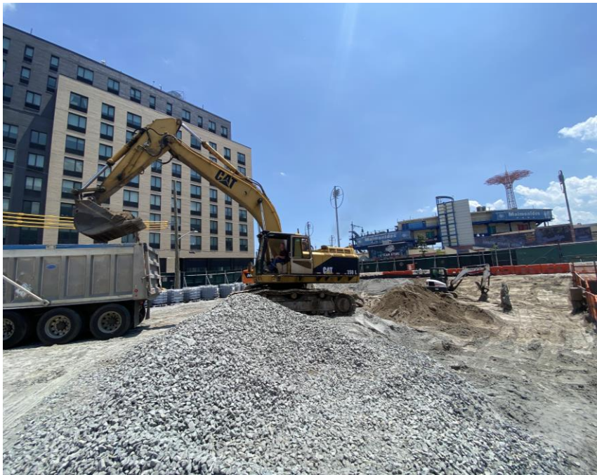
Photo 2: Precise loading non-hazardous fill/soil for offsite disposal in the southern part of the site (facing southeast).
