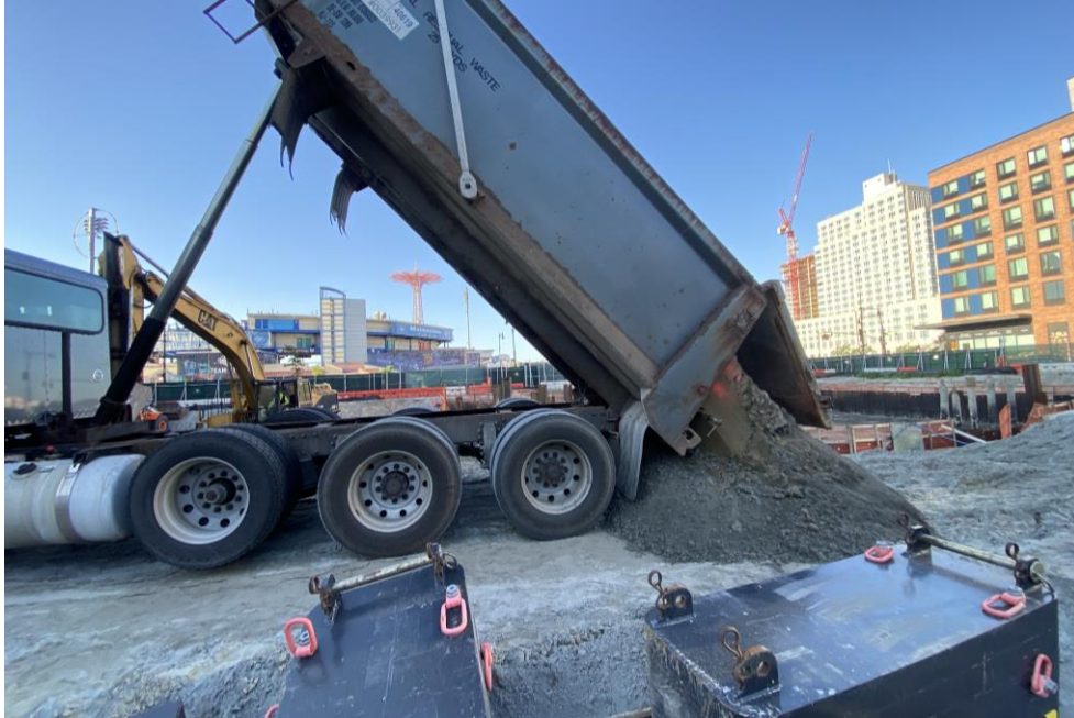
Photo 1: Precise importing pipe sand in the eastern part of the site (facing southwest).
