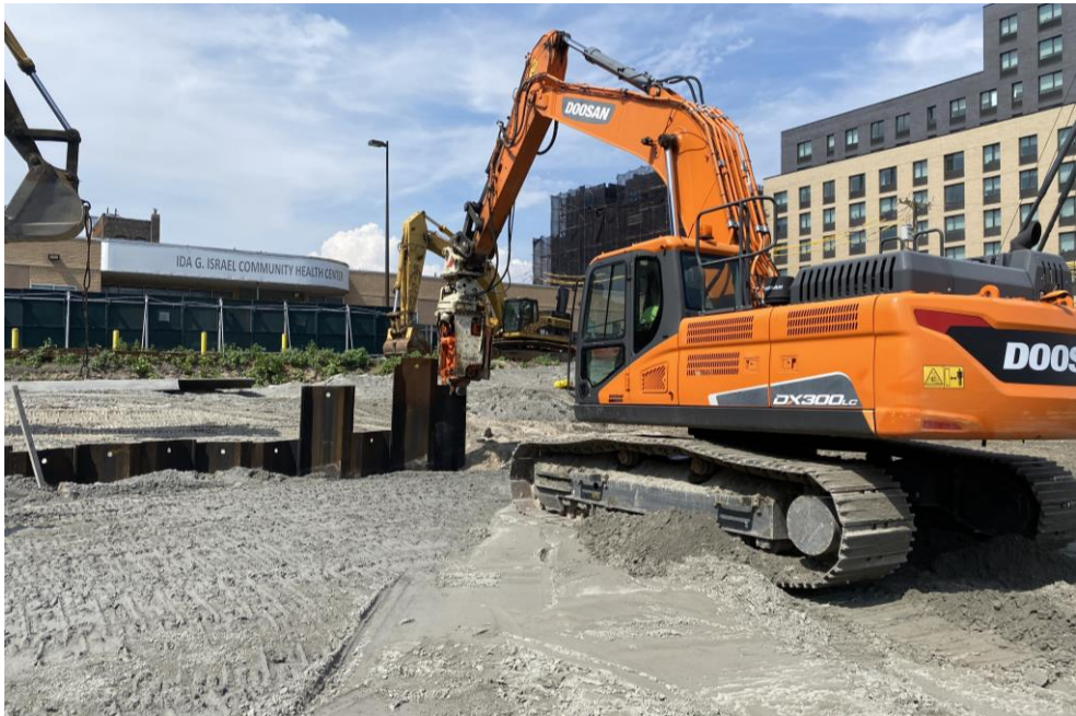
Photo 1: Precise removing sheet piles in the southern part of the site (facing northeast).
