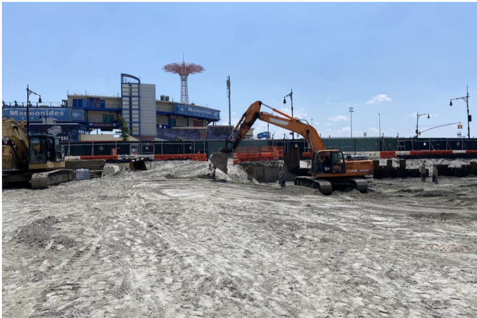
Photo 2: Precise grading pipe sand in the southern part of the site (facing south).
