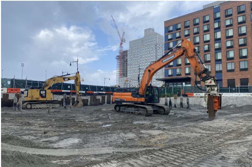
Photo 1: Precise removing sheet piles in the southern part of the site (facing southwest).
