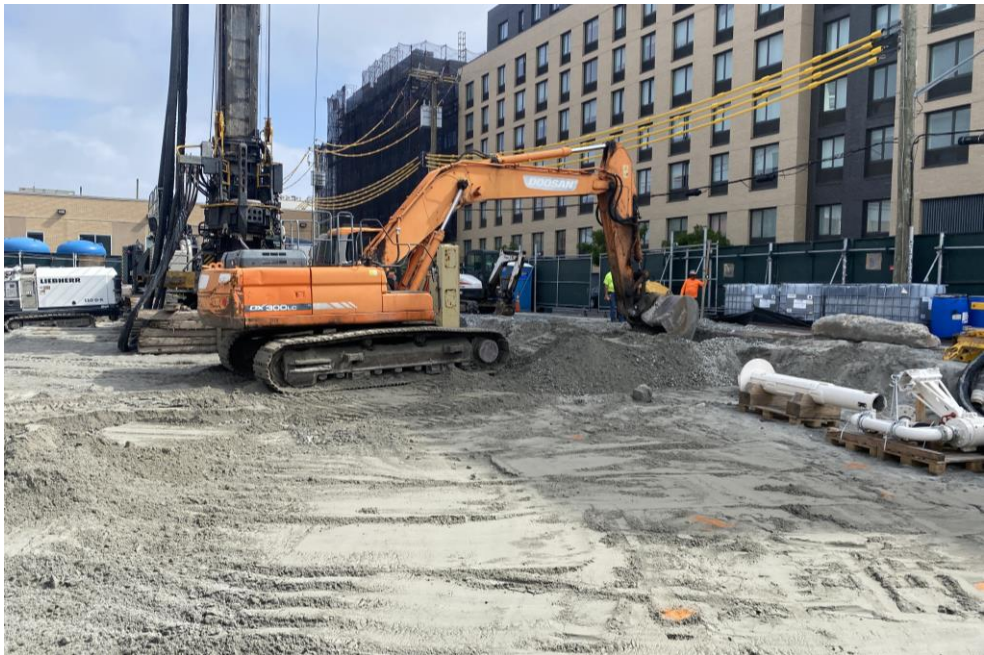
Photo 2: Precise excavating previously backfilled pipe sand in the eastern part of the site (facing northeast).
