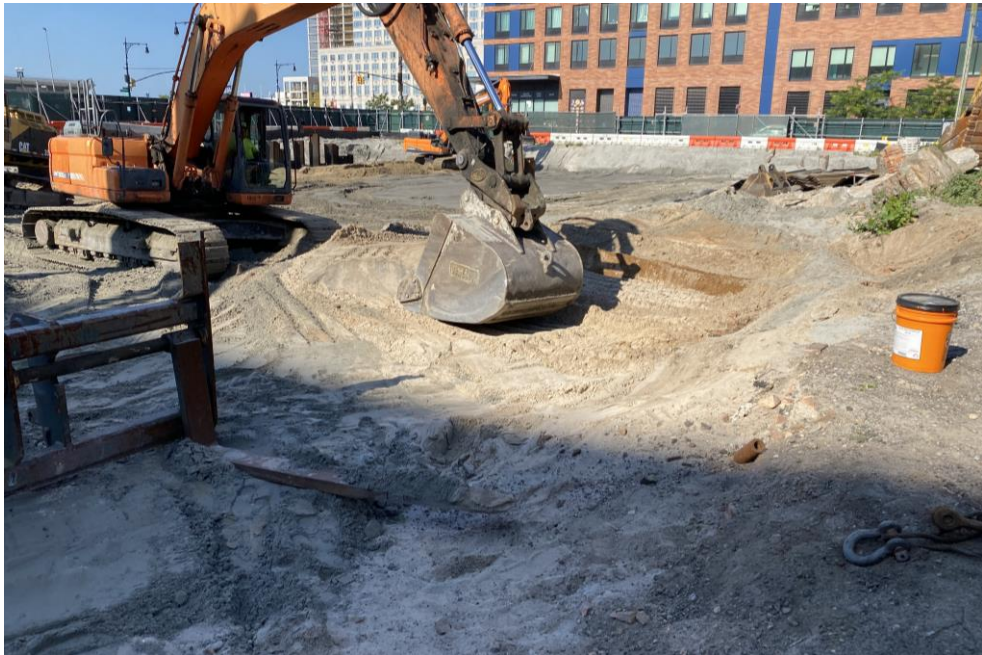
Photo 1: Precise grading in the central part of the site (facing southwest).
