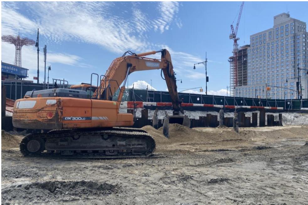
Photo 2: Precise backfilling pipe sand in the southern part of the site (facing south).
