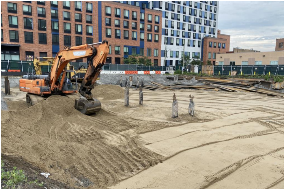
Photo 1: Precise grading pipe sand in the southern part of the site (facing northwest).
