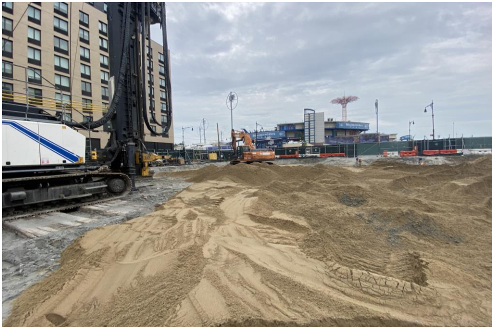
Photo 2: Precise backfilling pipe sand in the eastern part of the site (facing northeast).
