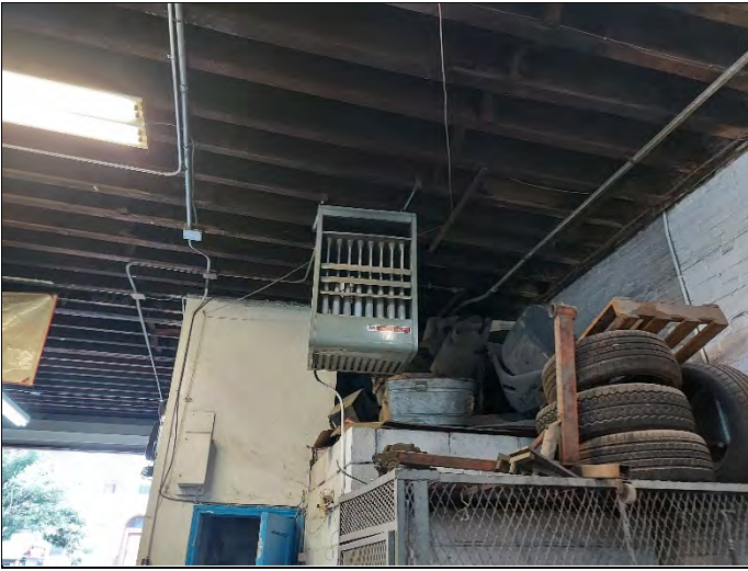
7. Ceiling-hung natural gas-fired blower
