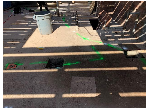
Image 11: Sewer is the only thing coming into the garage and it was marked in green.
