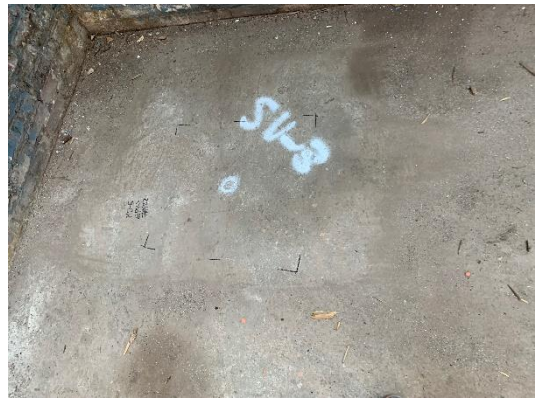
Image 7: This location had no utilities located and is clear for drilling
