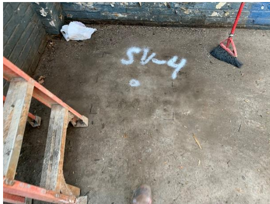
Image 8: This location had no utilities located and is clear for drilling
