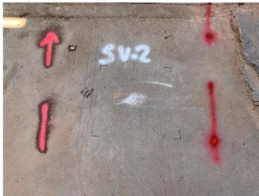
Image 3: This location was moved several times because of electrical lines that were located using EM scanner. The two conduits split off and it is safe to drill 2' off each electrical mark
