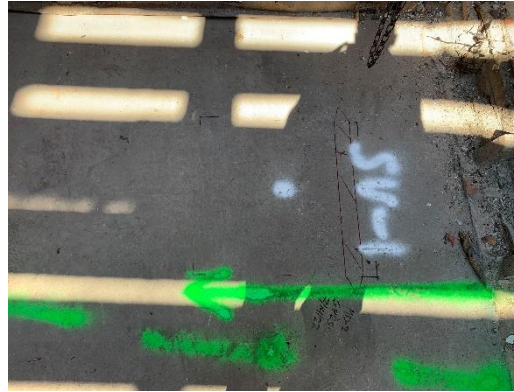
Image 1: This location had the conduit marked from data shot 1, as well as a sewer line that was located by direct connecting to the pipe inside of the cellar
