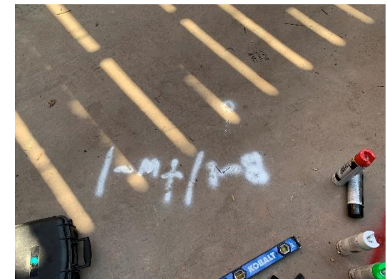
Image 2: This location had no utilities located and is clear for drilling
