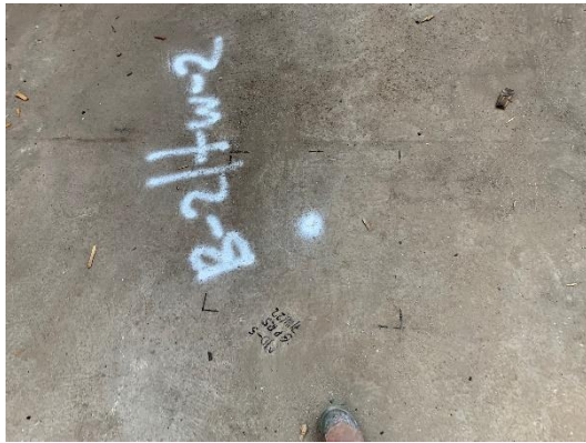
Image 6: This location had no utilities located and is clear for drilling
