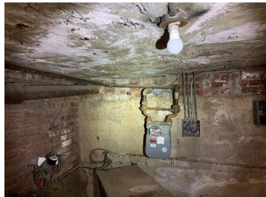
Image 9: Gas, water, electric and sewer all come into the cellar. Water is cut off here.
