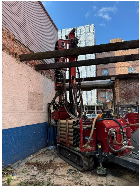
Photo 2: View of contractor installing soil vapor point SV-04 using a sonic drill rig, facing west.
