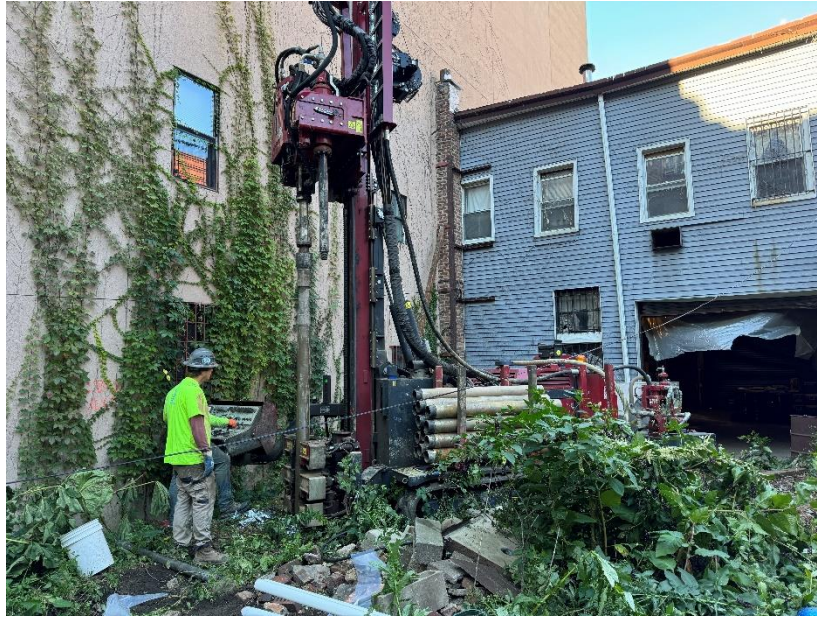
Photo 1: View of contractor installing monitoring well MW-05 using a sonic drill rig, facing southwest.
