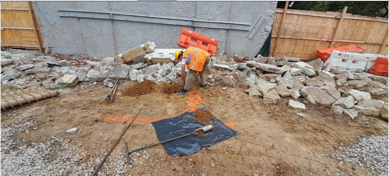
Photo 1: Trinity pre-clearing RXSB-8.
