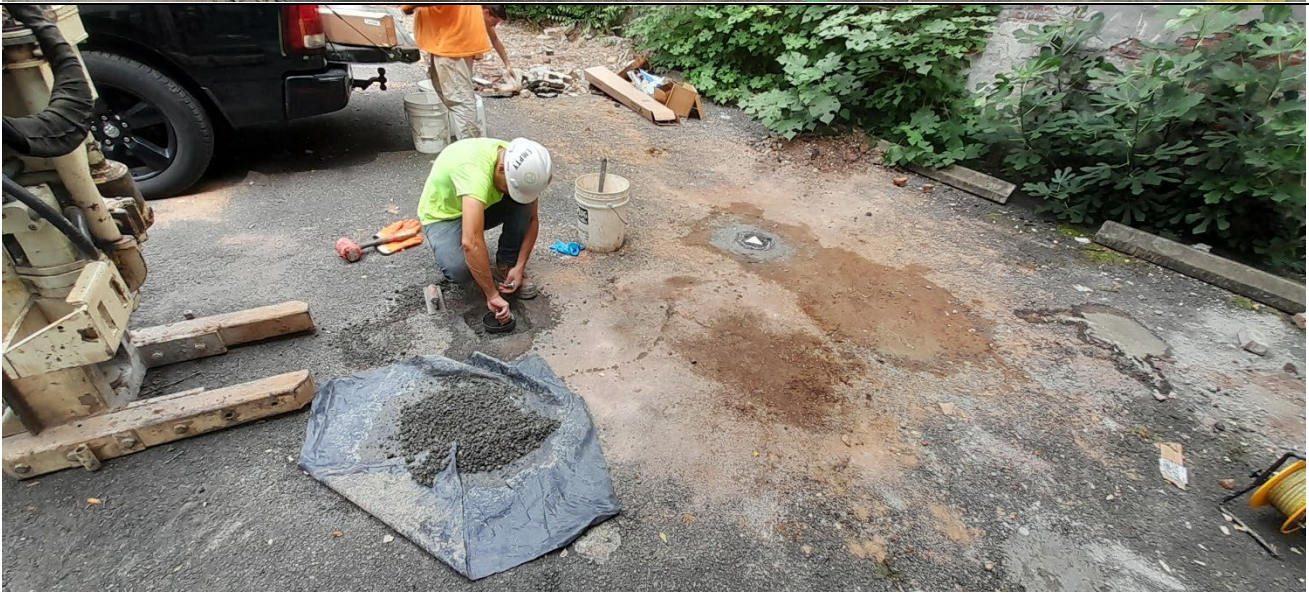
Photo 4: Trinity completing installation of RXSV-4.
