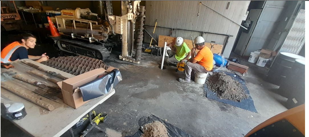
Photo 3: View of Trinity installing RXMW-12.
