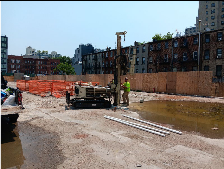
Photo 2: Looking southeast; view of Coastal advancing soil boring PDI-06.
