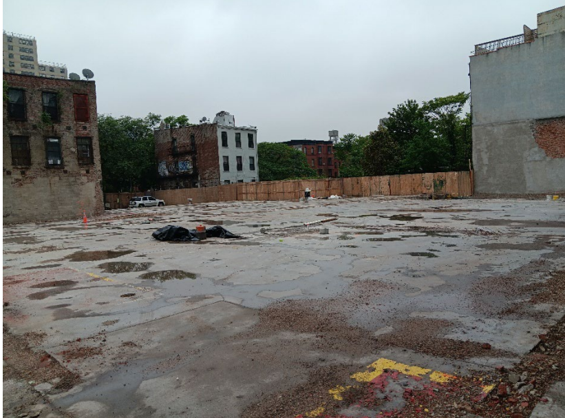
Photo 4: Looking southwest; view of general Site conditions.
