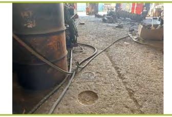
**Photo #11:** View of closed in place 1,080-gallon diesel UST within warehouse of the building.
