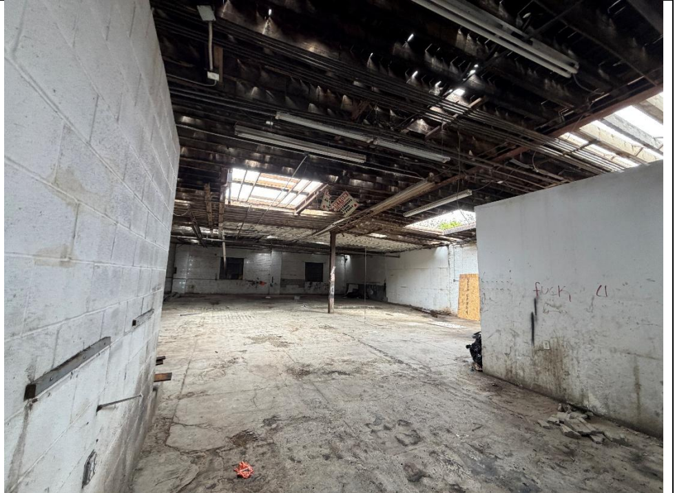
Photo 4- Asbestos removal and roofing status.
