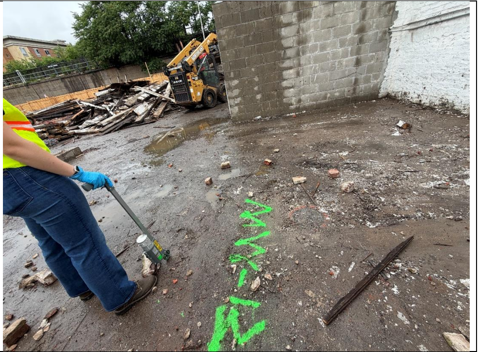
Photo 5 – View of BCP Site displaying location of MW13 on site post demolition.
