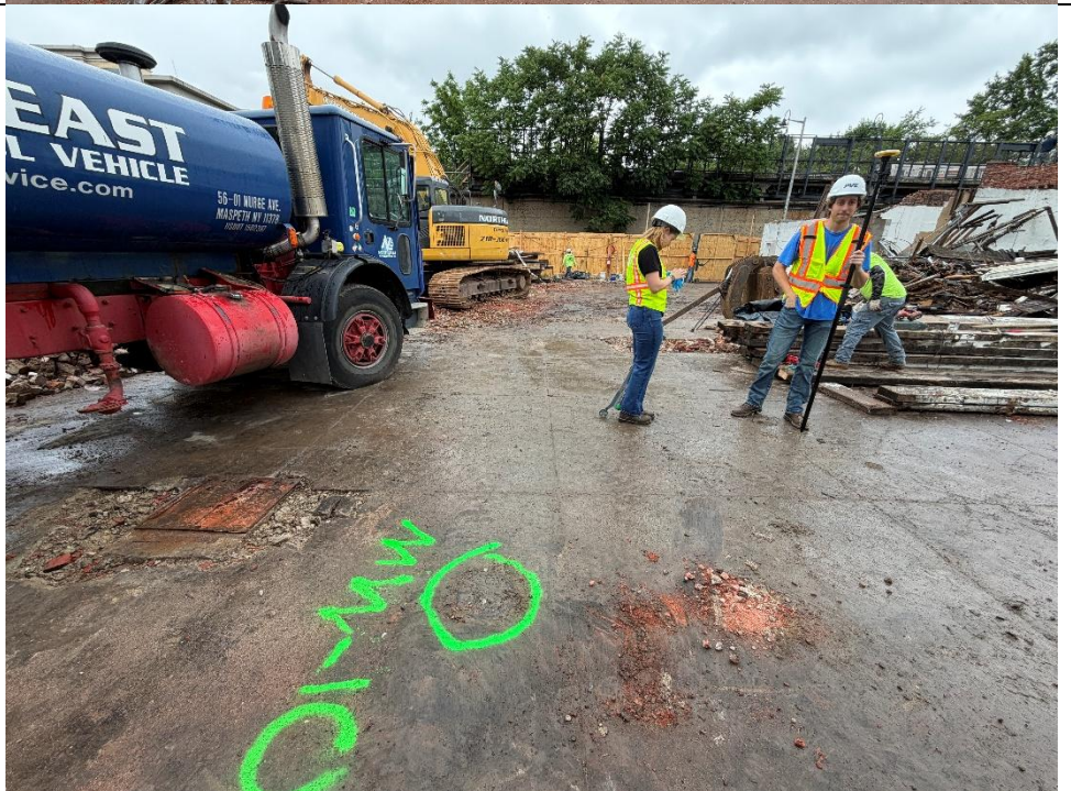
Photo 4 – View of BCP Site displaying location of MW10 on site post demolition.
