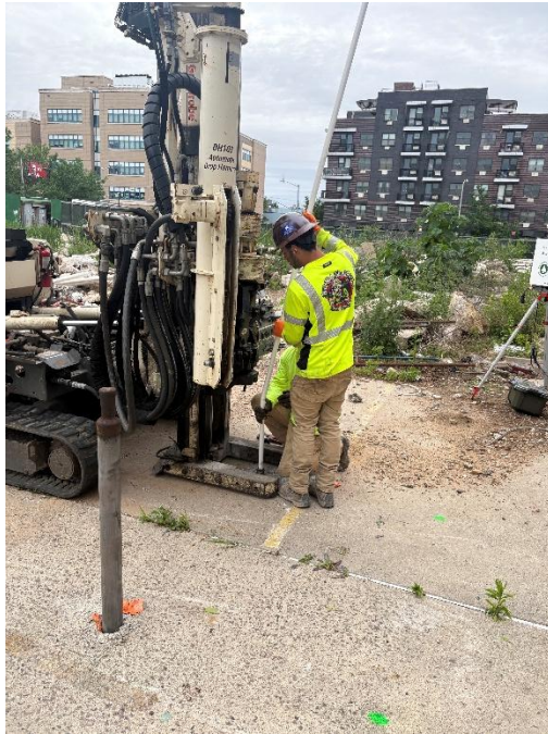
Photo 1: View of contractor installing monitoring point MP-3_10 along the eastern perimeter of the Site, facing northwest.
