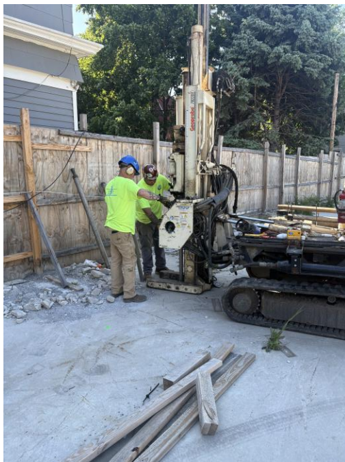
Photo 1: View of contractor installing SVE-1_Pilot test well along the eastern perimeter of the Site, facing southeast.
