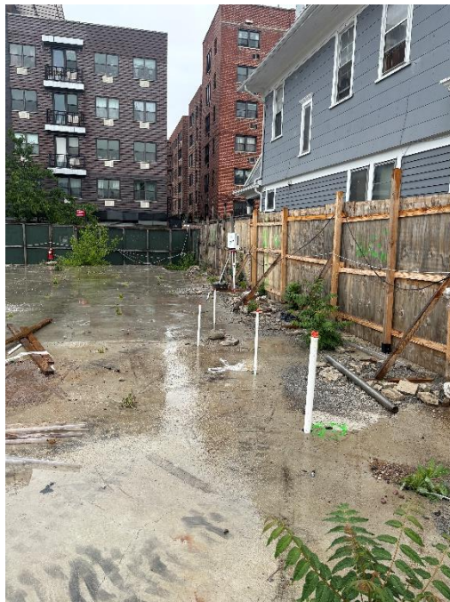
Photo 3: View of SVE-1_Pilot test area and AQS1/Receptor 1 CAMP station, facing north.
