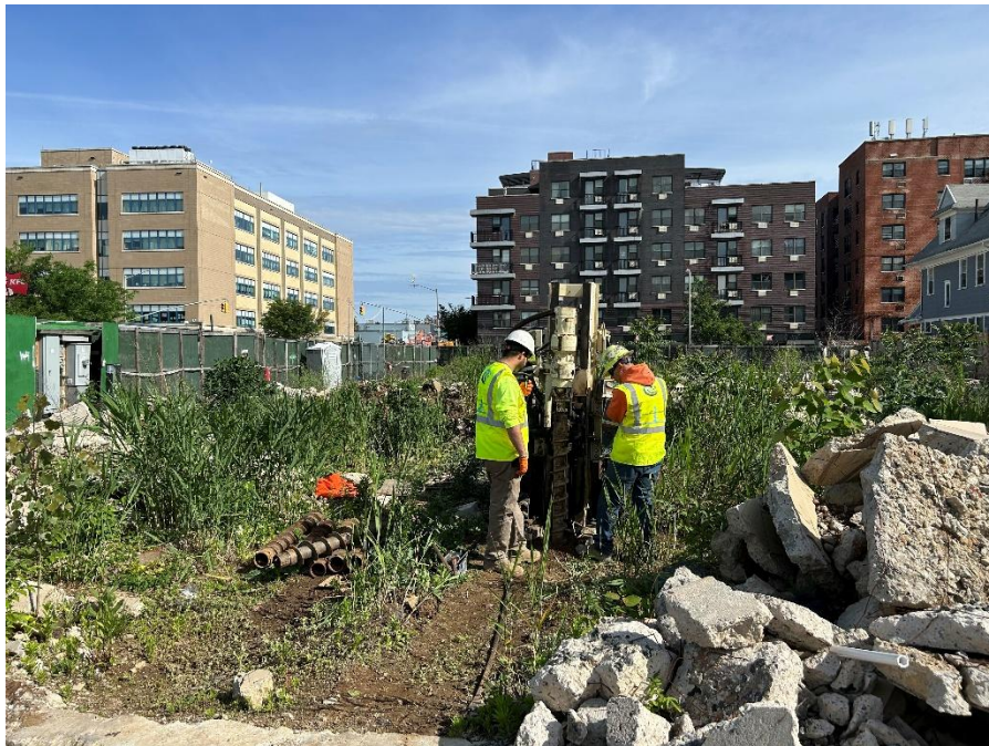
Photo 2: View of contractor drilling at the SVE-2_Pilot well location, facing north.
