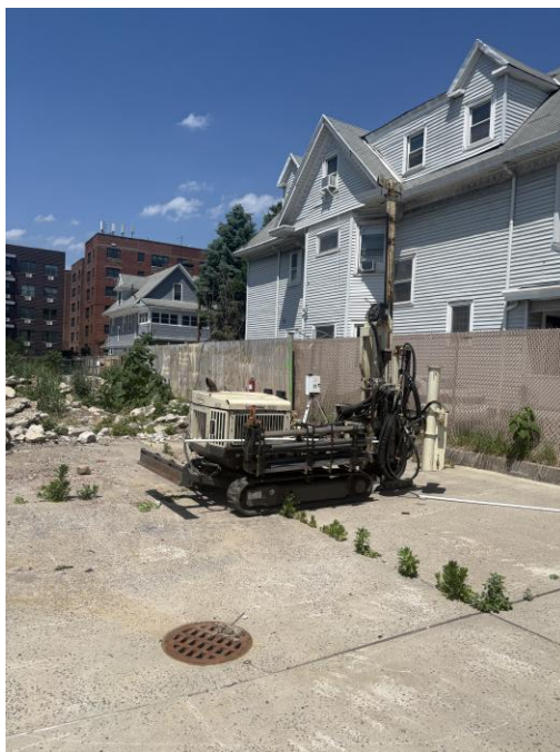
Photo 2: View of contractor installing monitoring point MP-3_15, facing northeast.
