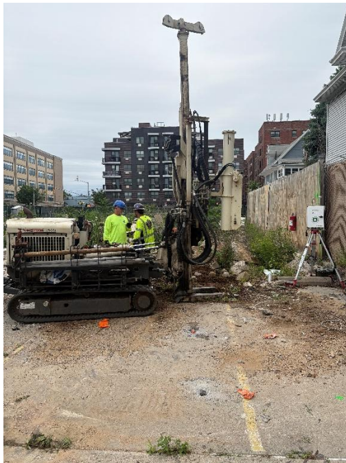
Photo 2: View of contractor installing SVE-3_Pilot well and AQS2/Receptor 2 CAMP station, facing north.
