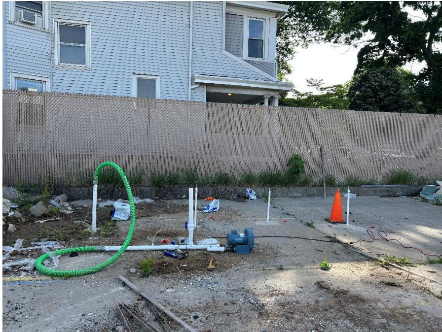
Photo 3: View of SVE-3_Pilot testing, facing east.
