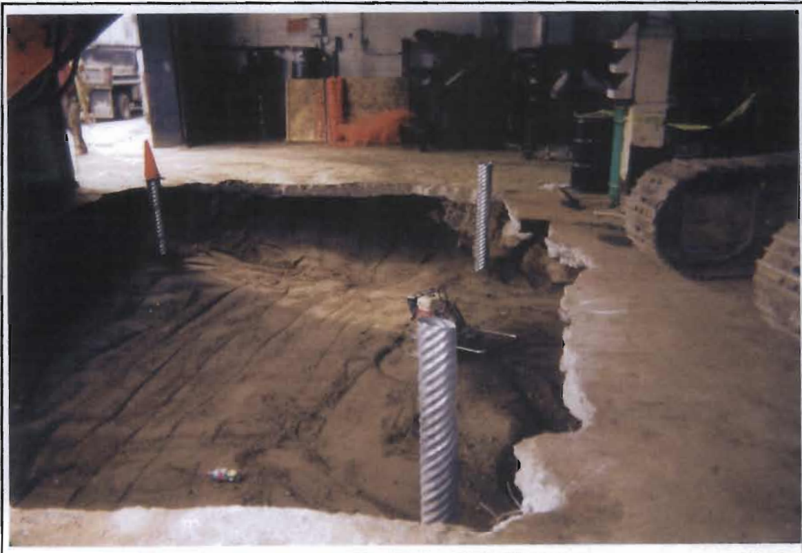
Photograph No.: 4 Date: 2/25/04 Description: Final site restoration.
