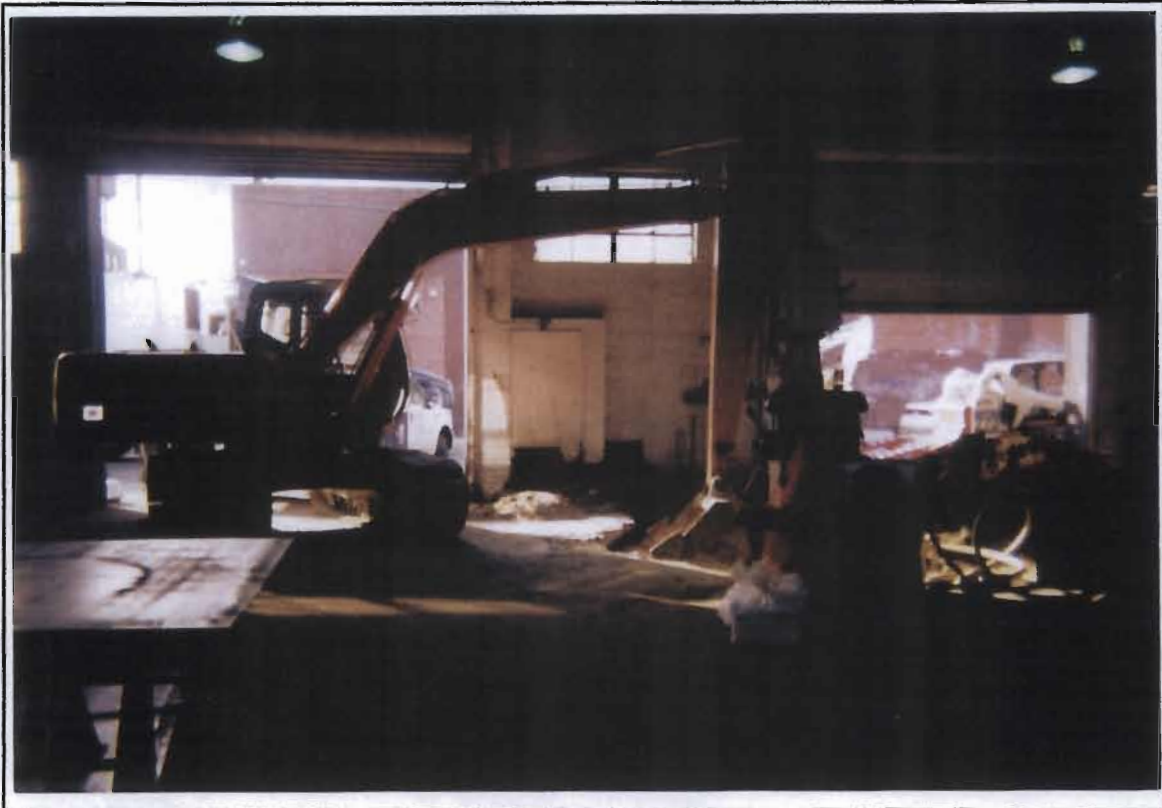
Photograph No.: 1 Date: 2/25/04 Description: Overall view of project location.
