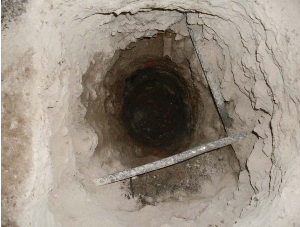
Photo 7- View of uppermost soil column at SB-SE-7 location. Note the reinforced concrete slab and the fraction of crushed red brick in the uppermost fill material.
