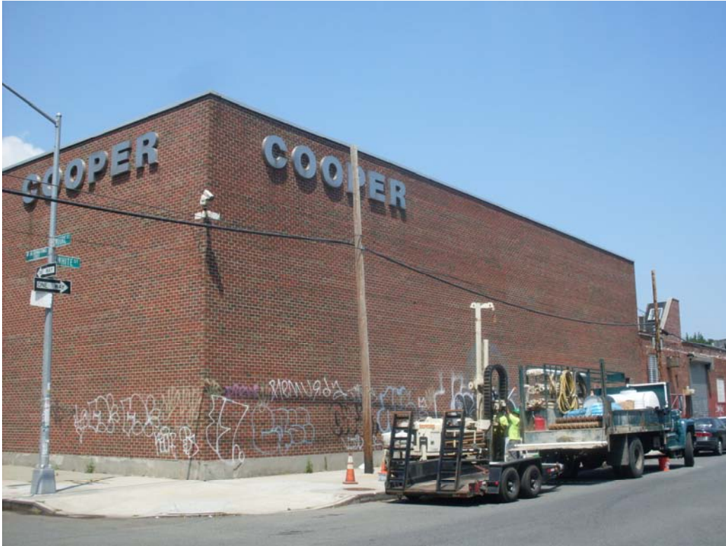
Photo 1- General investigation area- Northwest corner of Moore Street and White Street adjacent to Cooper Tank and Welding Corp.
