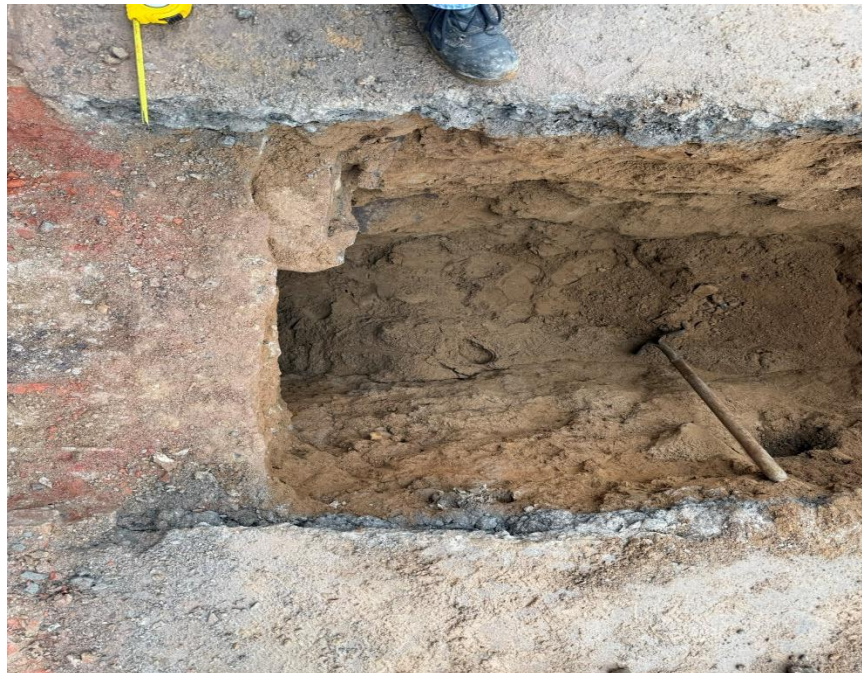
Photo 2: View of test pit in the southwestern part of the site
