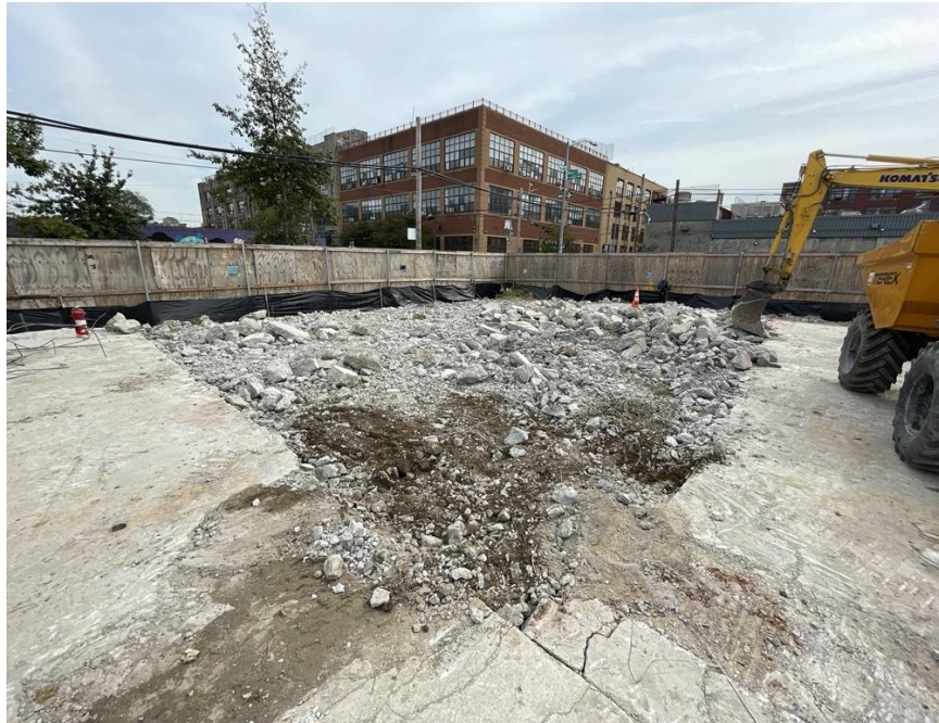
Photo 1: Kingdom demolishing the concrete slab in the southeastern part of the site (facing southeast)
