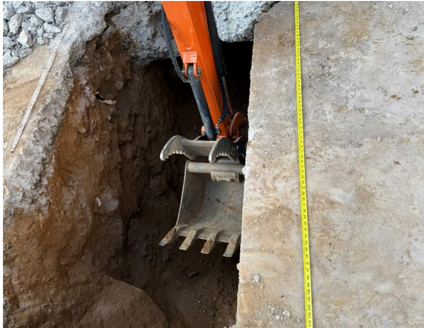
Photo 1: Wolf excavating a geotechnical test pit in the southwestern part of the site (facing west)
