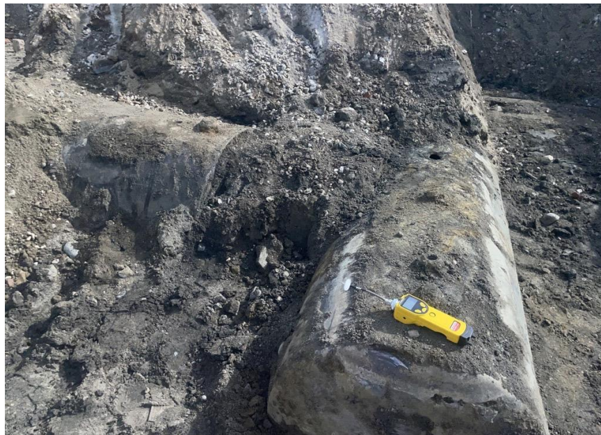
Photo 2: USTs uncovered in the southeastern part of the site (UST1 on right, UST2 on left) (facing south)
