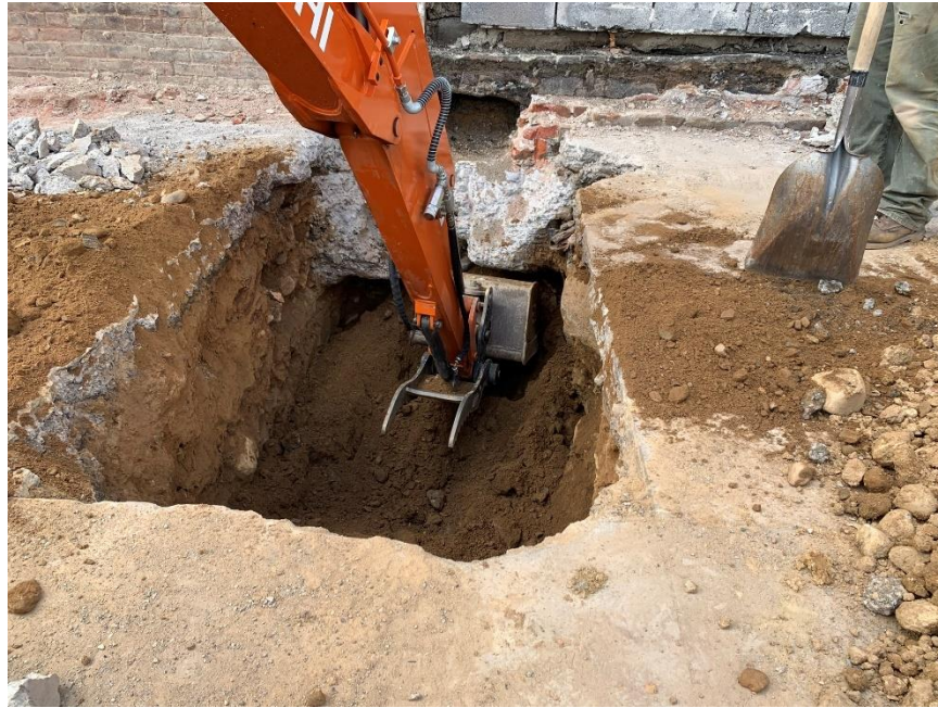
Photo 3: Wolf excavating a geotechnical test pit in the southwestern part of the site (facing west)
