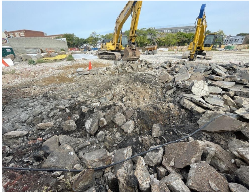
Photo 1: Kingdom demolishing the concrete slab in the southwestern part of the site (facing north)
