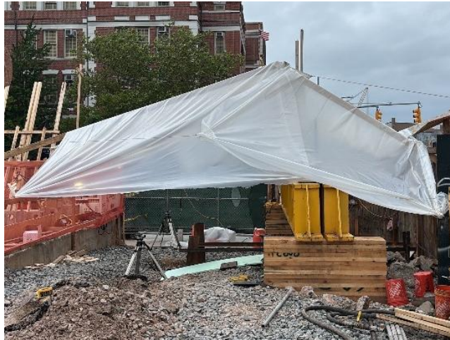
Photo 1: View of load test setup, facing west.
