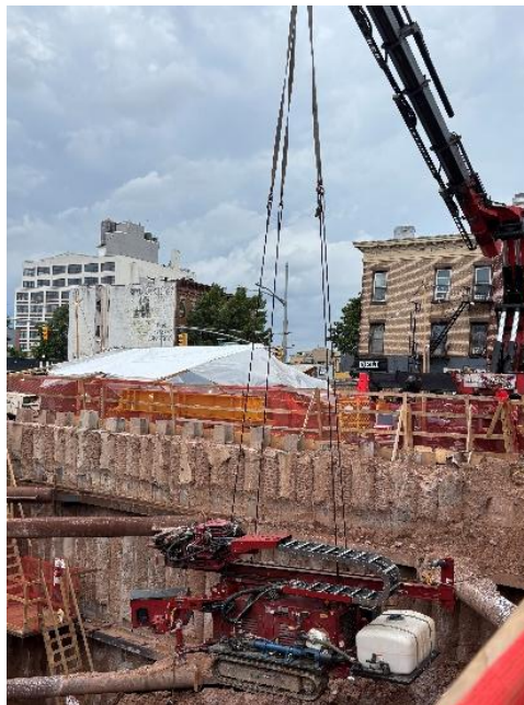
Photo 2: View of contractor lowering drill rig into the excavation, facing north.
