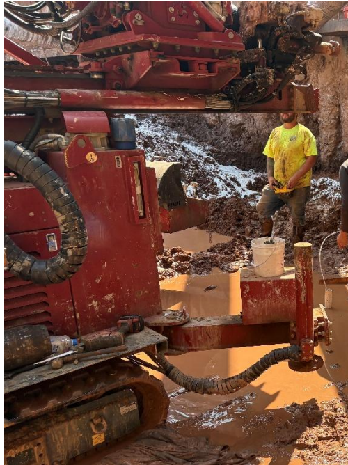
Photo 1: View of Coastal conducting drilling activities, facing east.
