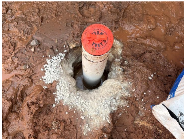
Photo 2: View of installed well, facing northwest.
