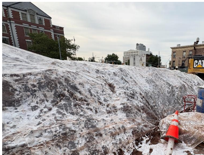
Photo 2: View of stockpile covered with foam and poly at end of day, facing northeast.
