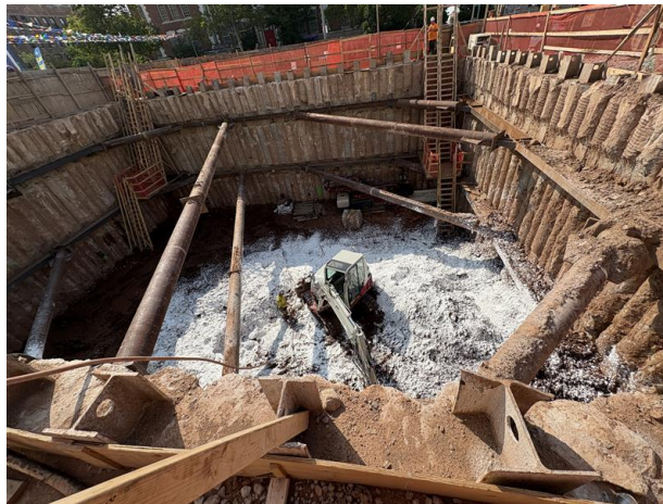
Photo 2: View of contractor applying odor suppressant at end of day on soil within the excavation, facing northwest.
