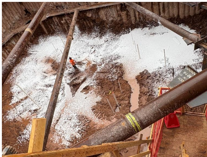
Photo 2: View of contractor applying odor suppressant at end of day on soil within the excavation, facing southeast.
