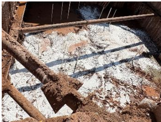
Photo 2: View of contractor applying odor suppressant at end of day on soil within the excavation, facing southwest.
