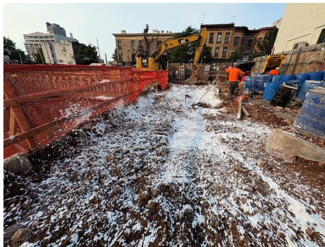
Photo 2: View of contractor applying odor suppressant at end of day on soil within the former stockpile area, facing northeast.
