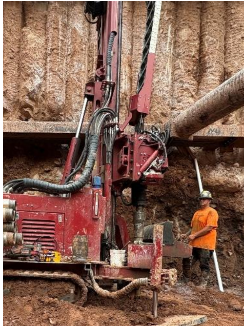
Photo 1: View of Coastal conducting drilling activities, facing southeast.
