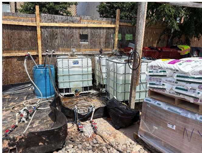
Photo 2: View of Isotec performing ISCO injections pilot test at IW-9, facing northeast.
