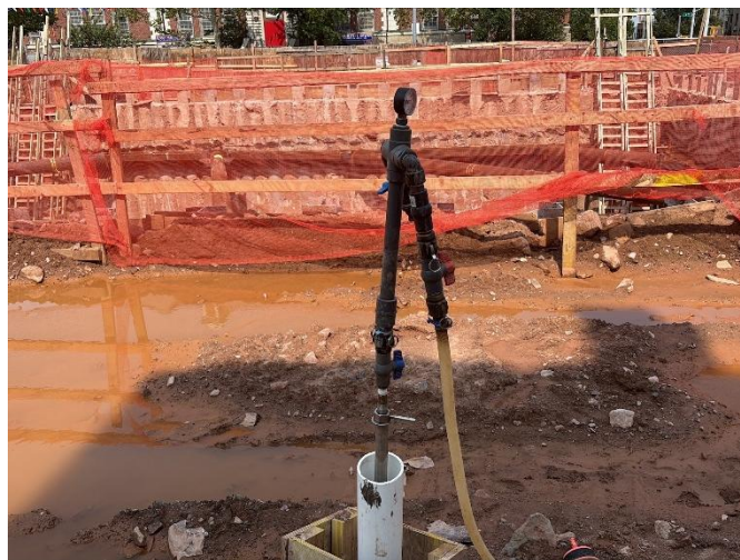
Photo 2: View of Isotec performing ISCO injections pilot test at IW-6, facing north.
