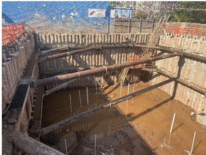
Photo 2: General site view, facing north.
