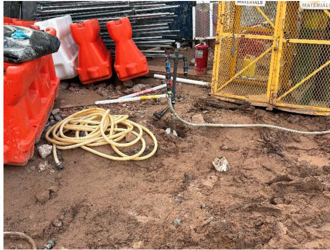
Photo 1: View of Isotec performing ISCO injections pilot test at IW-3, facing northeast.
