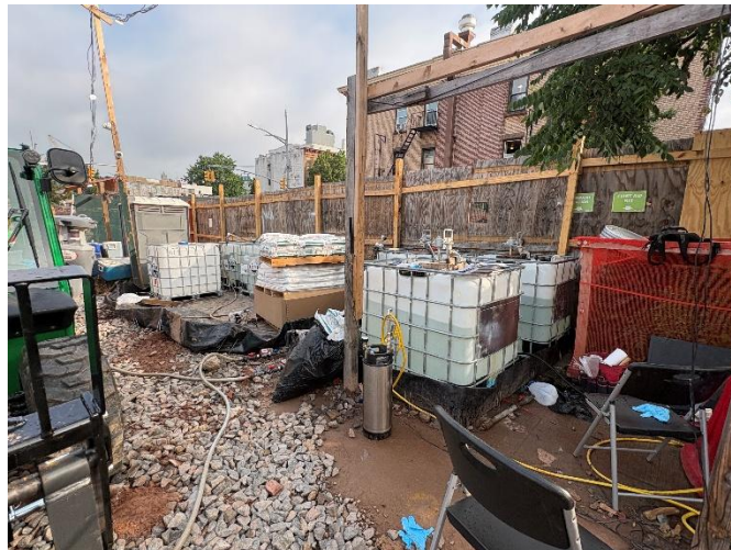
Photo 2: View of Isotec performing ISCO injections pilot test at IW-9, facing north.
