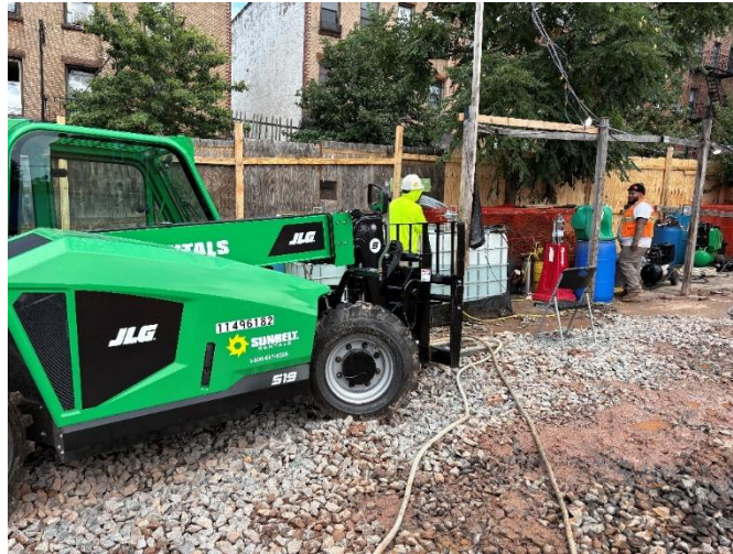
Photo 1: View of Isotec setting up for the ISCO injections pilot test, facing southeast.
