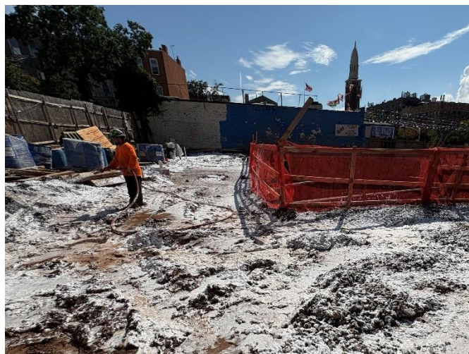
Photo 2: View of contractor applying odor suppressant at end of day on soil, facing northwest.
