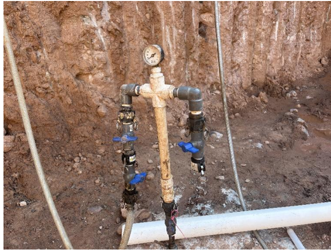
Photo 1: View of Isotec performing ISCO injections pilot test at IW-1, facing northeast.
