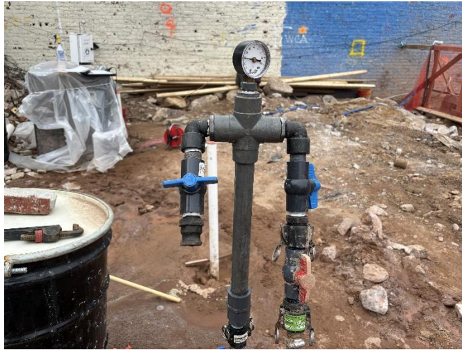
Photo 1: View of Isotec performing ISCO injections pilot test at IW-9, facing southwest.
