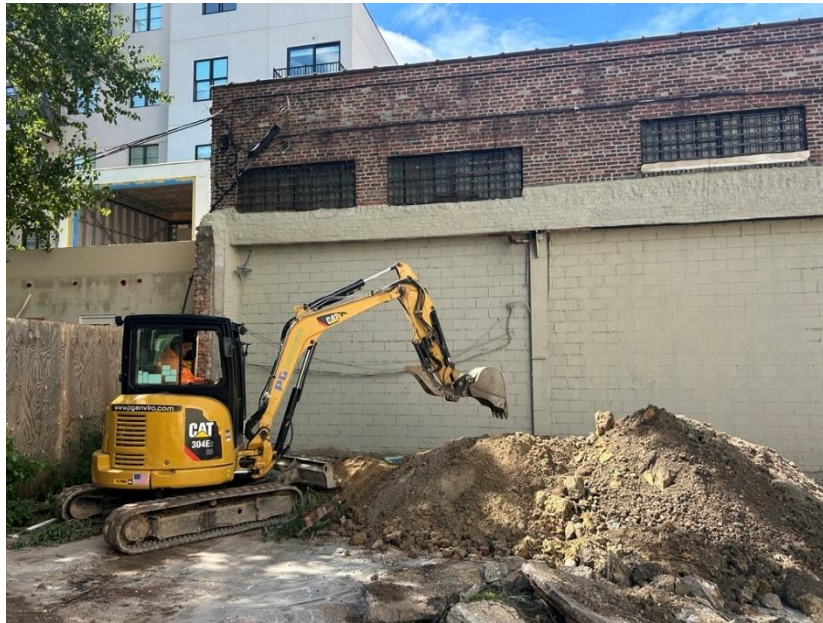
Photo 2: View excavating test pits, facing northwest.
