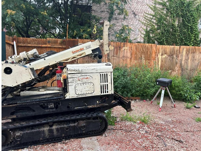
Photo 1: View contractors installing soil boring, facing northeast.
