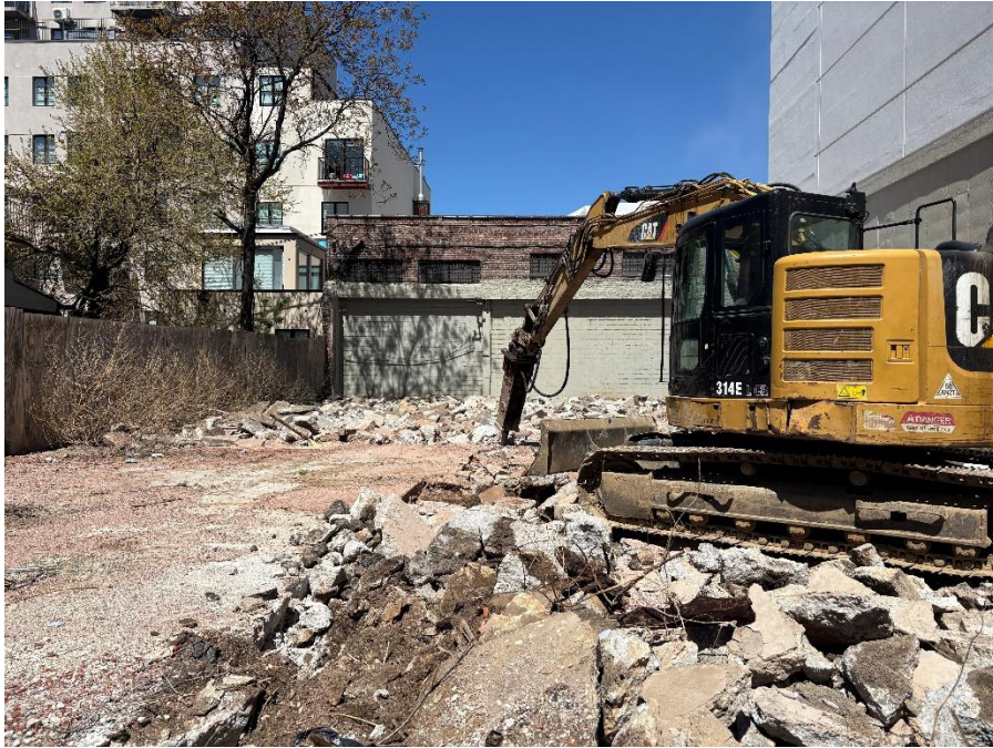
Photo 1: View of concrete demolition, facing northwest.
