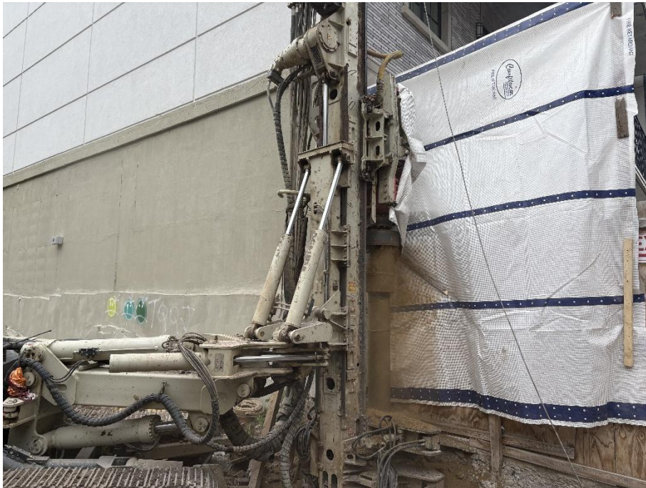
Photo 2: View of contractors drilling pile caps, facing north.
