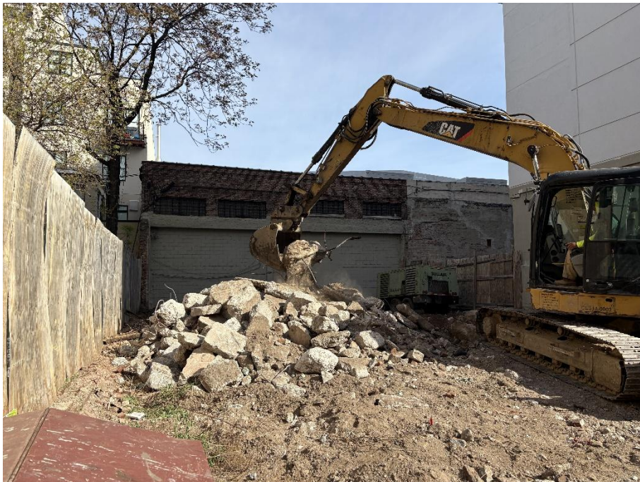
Photo 2: View of contractors excavating concrete from existing footings, facing northwest.
