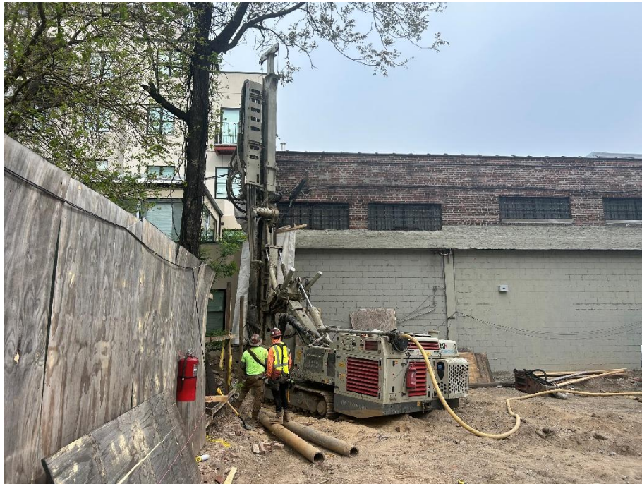
Photo 1: View of contractors installing soldier piles for SOE, facing north.
