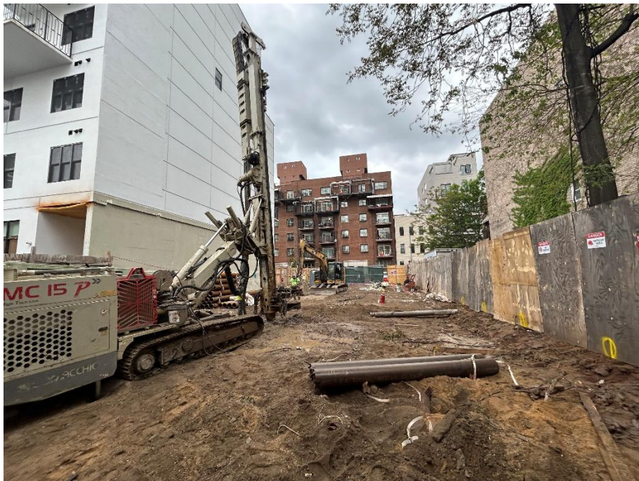
Photo 1: View of contractors installing soldier piles for SOE, facing north.
