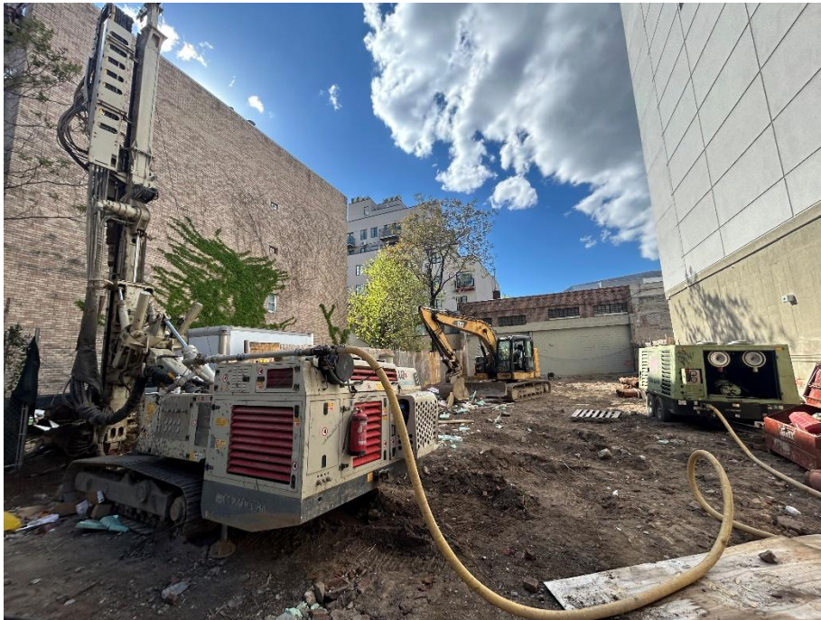
Photo 2: View of contractors installing soldier piles for SOE, facing northwest.
