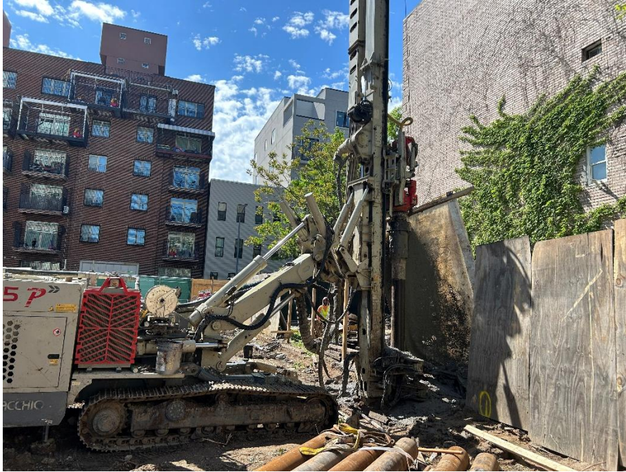
Photo 1: View of contractors installing soldier piles for SOE, facing southwest.
