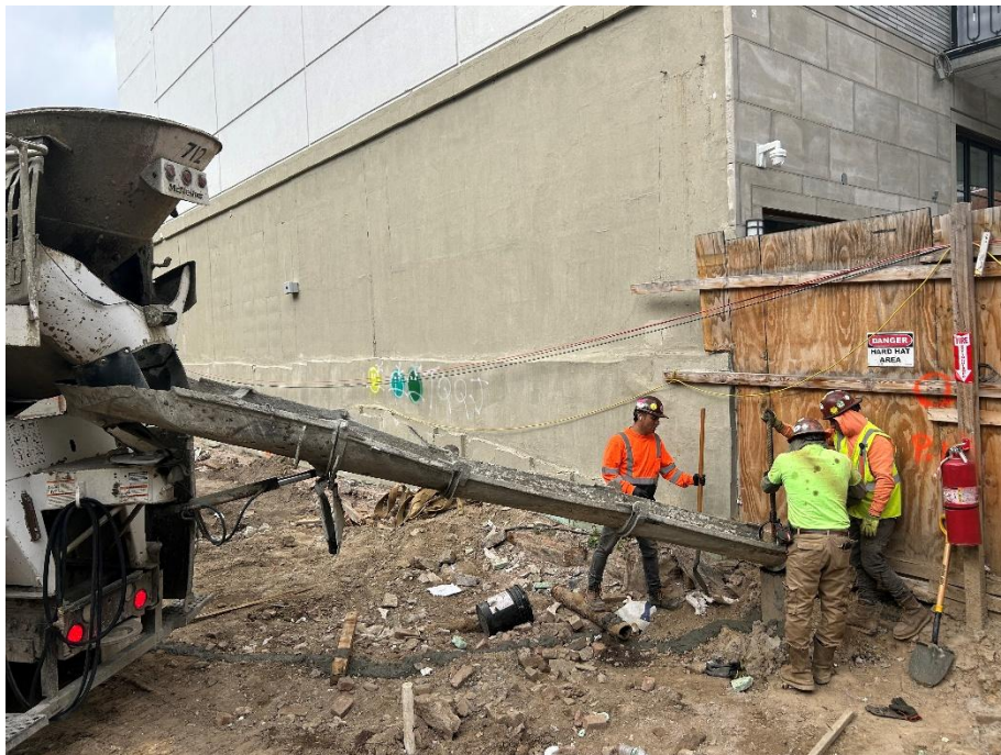
Photo 2: View of contractors grouting soldier piles, facing northeast.
