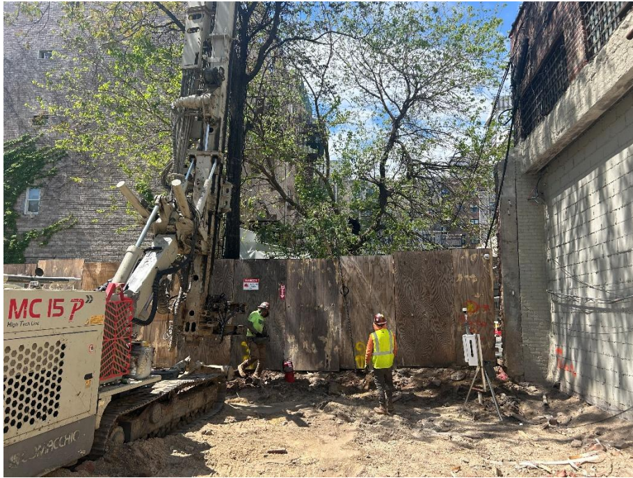
Photo 1: View of contractors reinforcing soldier piles with rebar, facing west.
