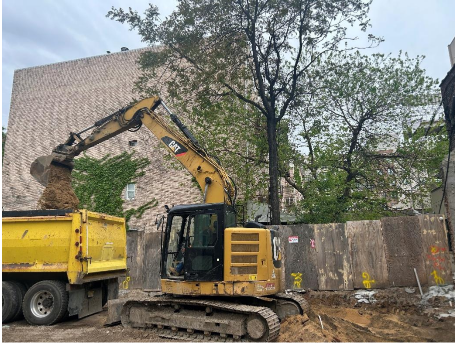
Photo 1: View of contractors loading tri-axle truck with soil/fill material, facing west.
