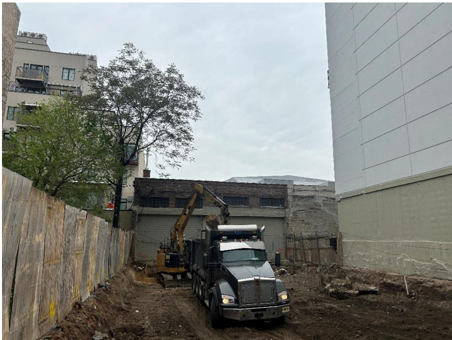
Photo 2: View of contractors loading tri-axle truck with soil/fill material, facing north.
