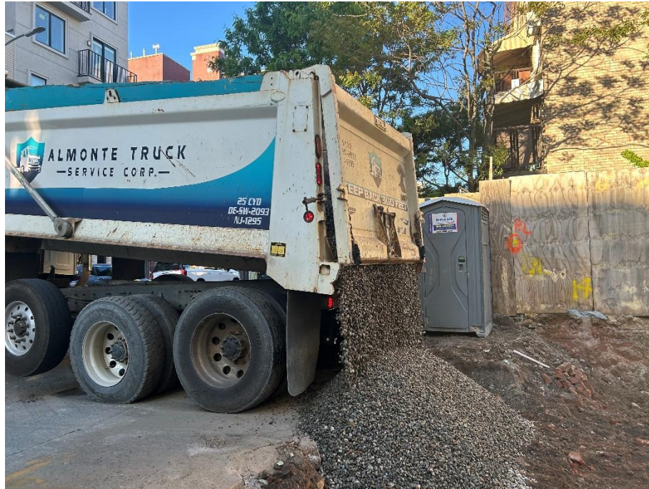
Photo 1: View of contractors importing \frac{3}{4} " ASTM #57 virgin stone, facing west.
