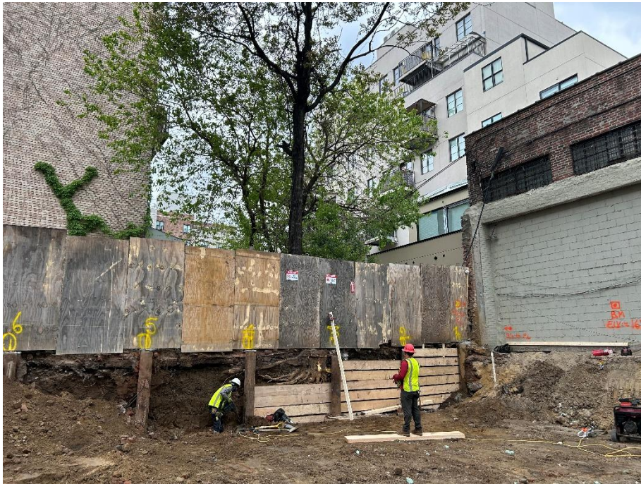
Photo 2: View of contractors installing timber lagging for SOE, facing northwest.
