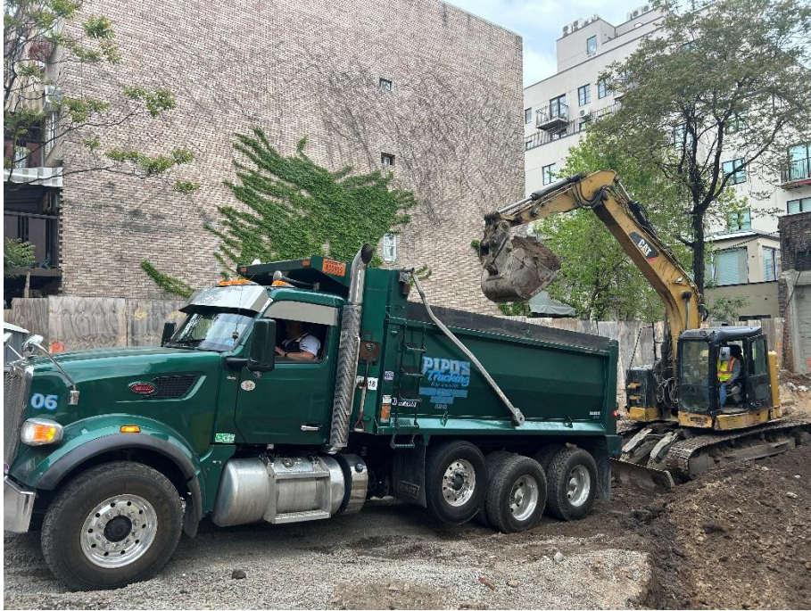
Photo 1: View of contractors loading tri-axle truck with soil/fill material, facing northwest.
