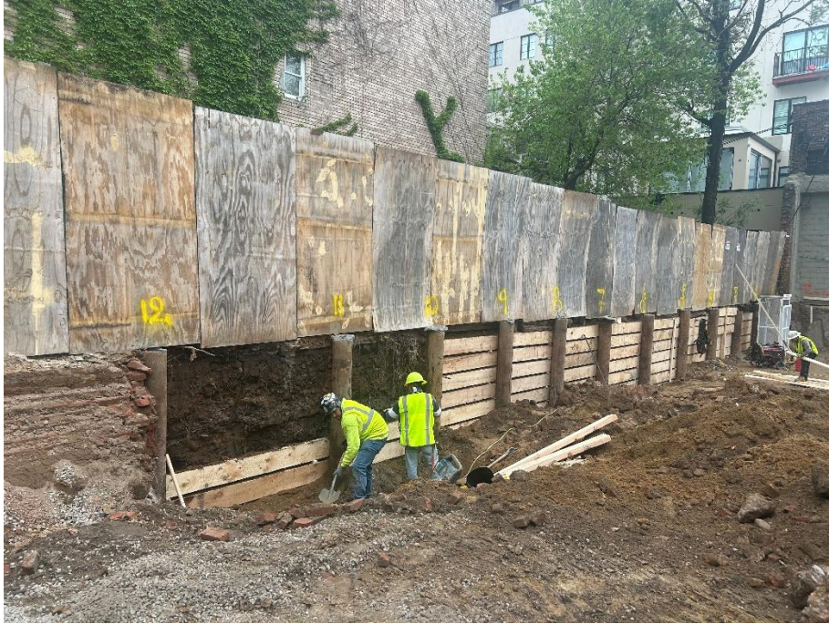
Photo 1: View of contractors installing timber lagging for SOE, facing northwest.
