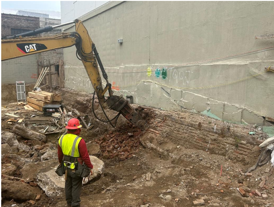
Photo 2: View of contractors removing C&D materials, facing northeast.
