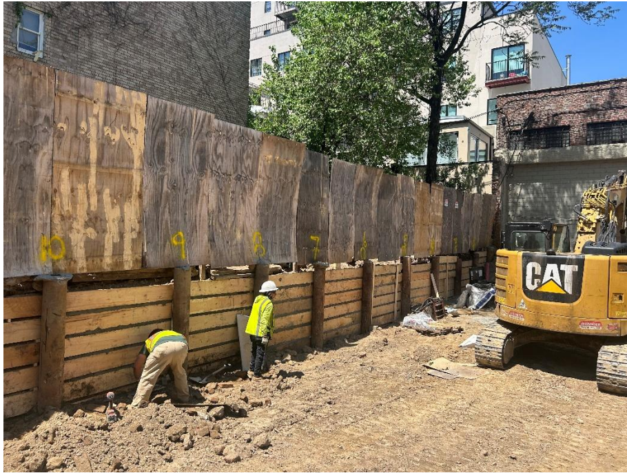
Photo 1: View of contractors installing lagging for SOE, facing northwest.
