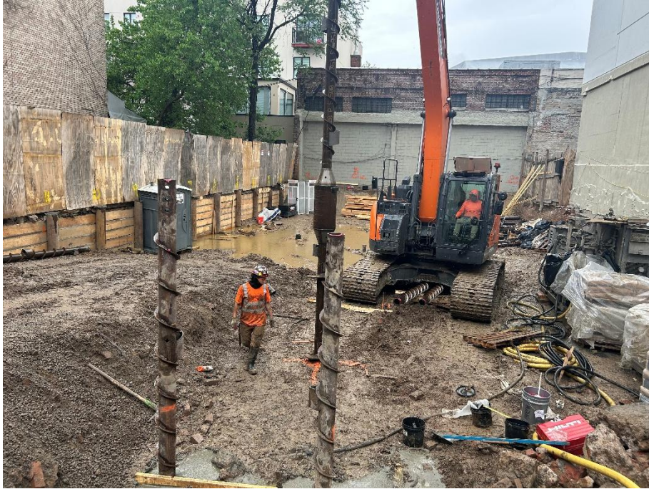
Photo 1: View of contractors installing auger cast piles, facing northwest.
