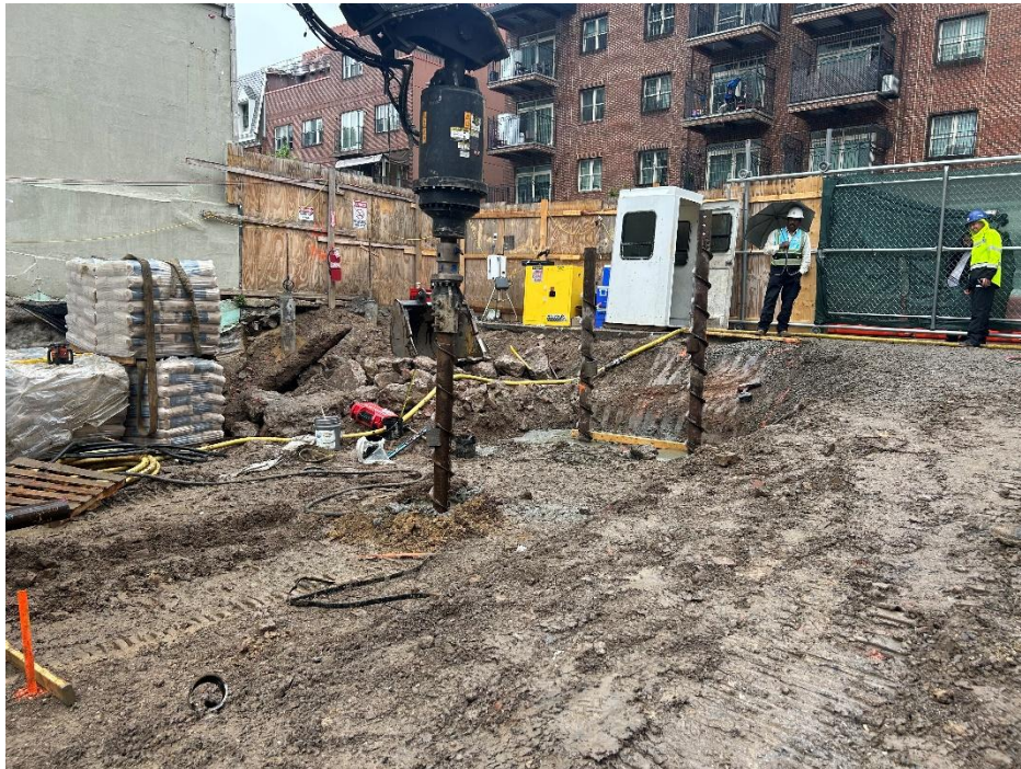
Photo 2: View of contractors installing auger cast piles, facing southeast.
