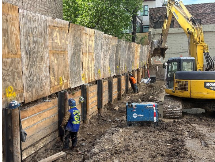
Photo 1: View of contractors welding steel beams, facing north.
