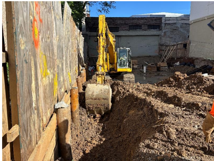
Photo 2: View of contractors preparing Site for welding, facing north.
